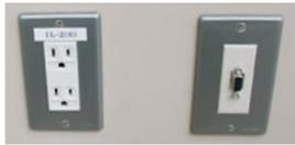
A PC input port (right) is installed in the classroom so PCs do not have to be permanently installed, thereby reducing security concerns.
